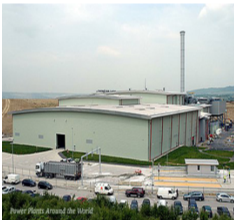
Fig. 3 – WTE Plant Kent UK .Photo Jan 2007
