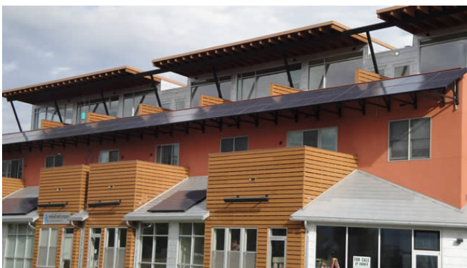
Fig.4 – Solar panels integrated into the design of the commercial property in Colorado.2009
