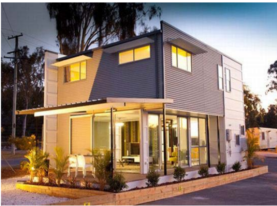
Fig 2 – “Green” Townhouses, Australia (Designer – Brett Blacklow) implementing sustainable energy efficient standards and extensive use of recycled materials
