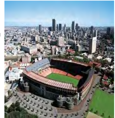
Fig 4: The completed soccer city stadium, one of the venues of FIFA world cup in South Africa. The project was an example of a successful project delivered with efficient PM expertise
